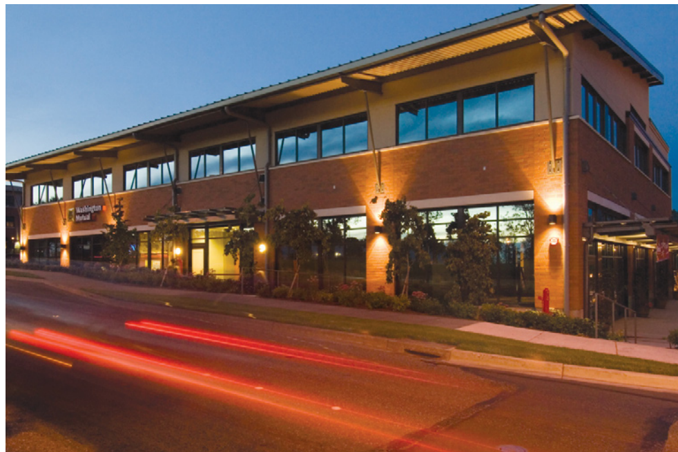
The Dahlia Building, on Barkley Boulevard, is home to a Washington Mutual branch, offices for Olympic Health Management, retail stores and a real estate office.
